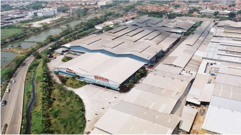
Kapuk Plant (Radiator Facilities)
